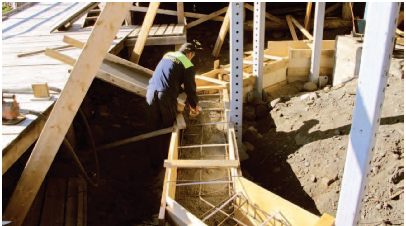
Fig. 2. Grouting of reinforced concrete foundation (underground part)
