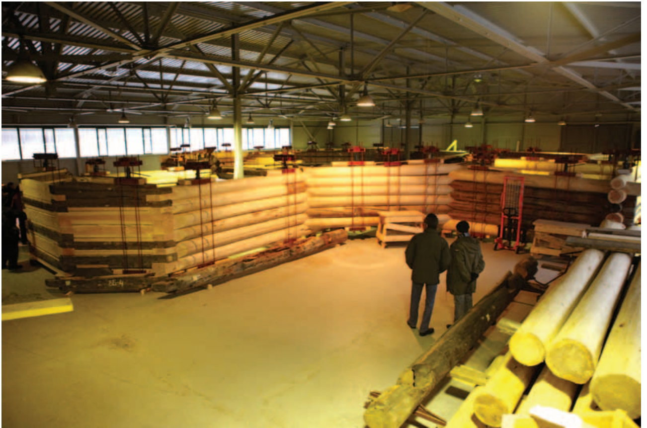
Fig. 13. Foundation after the restoration with applied load on the framework timber sets
