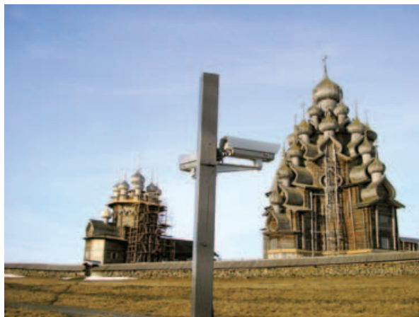
Fig.1. Sensors of infrared monitoring system mounted around the Kizhi Pogost
