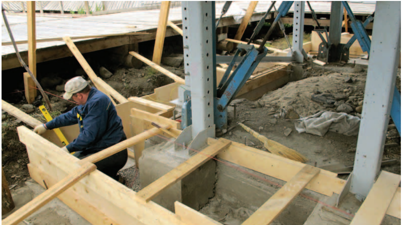
Fig. 1. Mounting of curb for grouting of reinforced concrete foundation (underground part)
