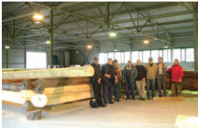
Fig. 13. Start of the basement framework assembly in the restoration assembly workshop
