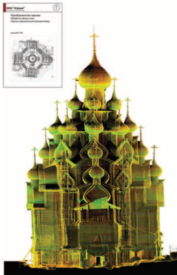
Fig. 3. 3D model developed as a result of laser scanning of the Church of the Transfiguration in 2010-2011
