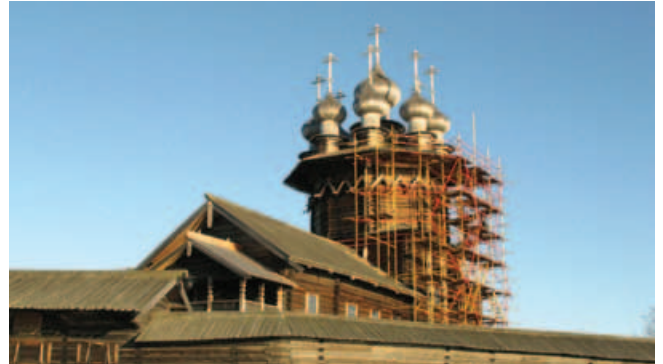
Fig. 22. Scaffoldings mounted for completion of roof restoration
