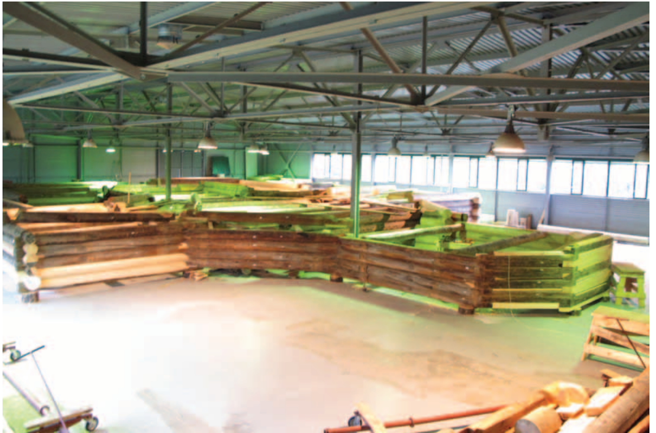
Fig. 11. Process of framework assembly
