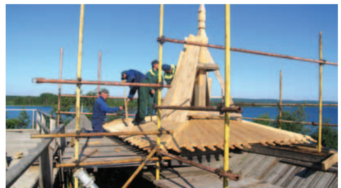
Fig. 23. Restoration of the northern tower of the Pogost enclosure
