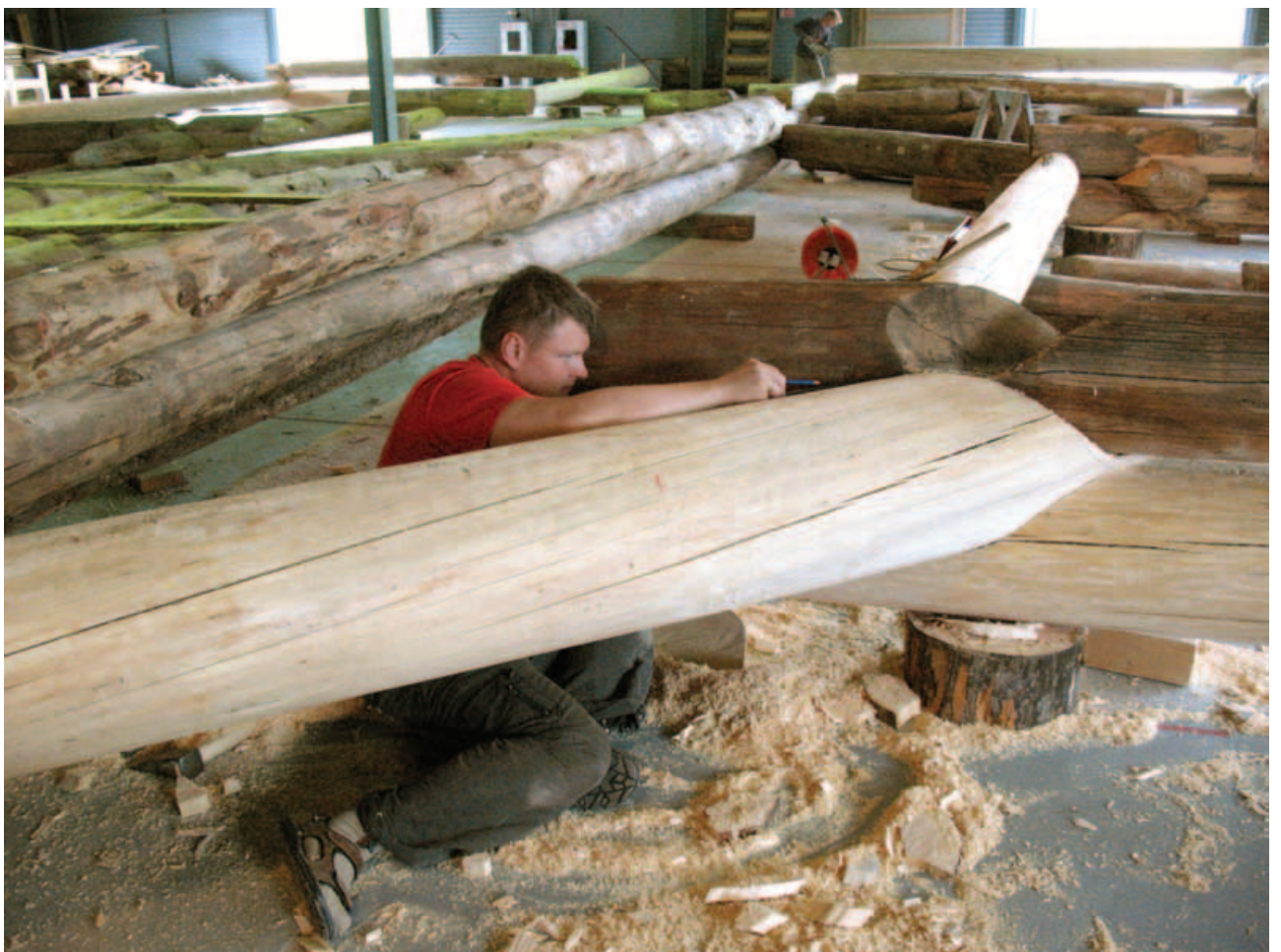
Fig. 10. Work on accurate superposition of historic and new wood in the monument framework
