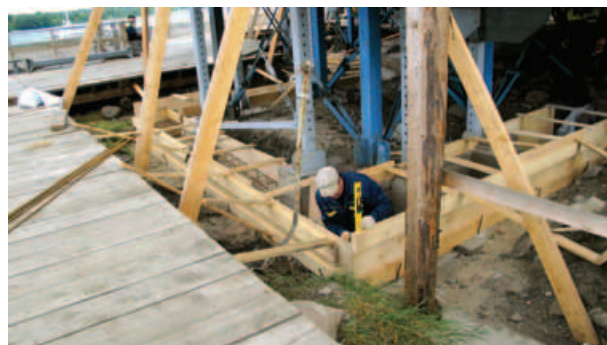
Fig. 7. Mounting of curb for underground part of the foundation
