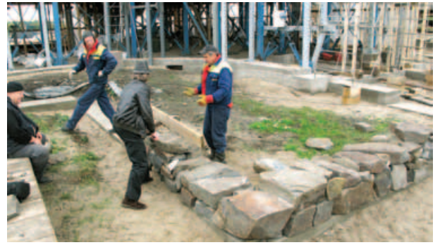
Fig. 9. Pilot part of loose rock foundation (above ground)
