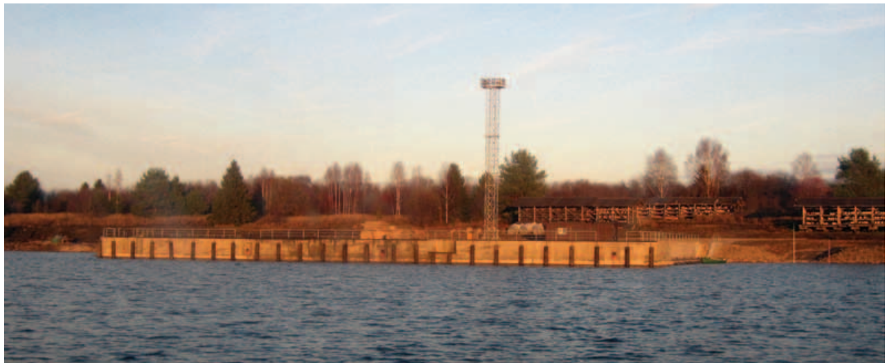
Fig. 6. New cargo terminal on Kizhi
