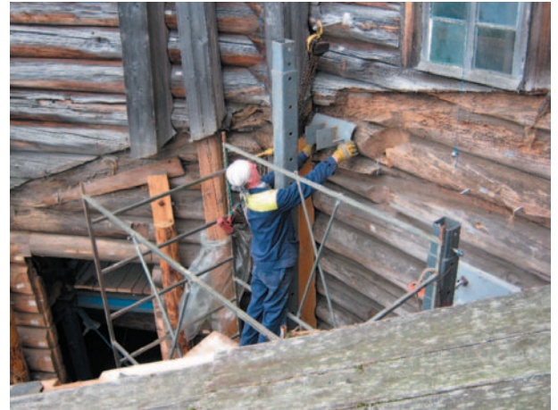
photo 4. Installation of lifting equipment.
