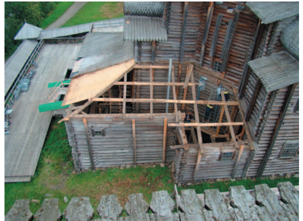
photo 9. The disassembly of the refectory in progress.
