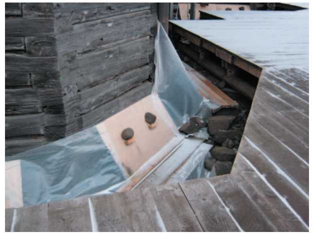
photo 11. Conservation of the foundation posts.
