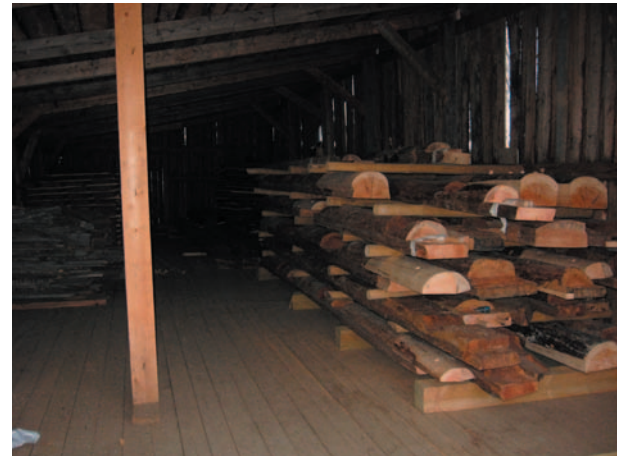
photo 8. The restored floor components are stockpiled before the restoration on Pogost.
