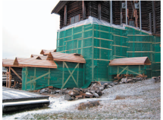
photo 10. The refectory after the disassembly.
