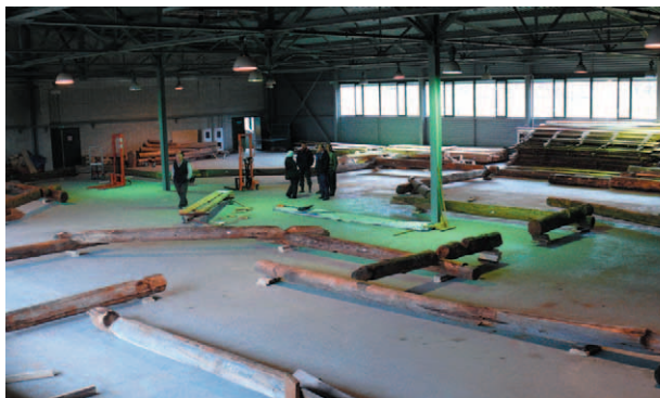
Fig. 30. Start of test-assembly of the restoration tier in the Restoration complex
