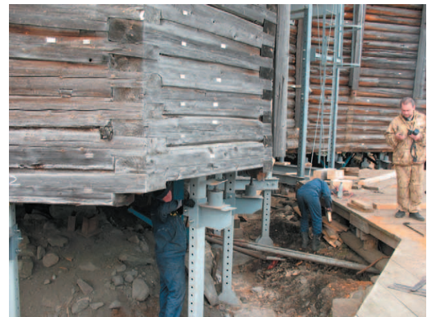
Fig. 25. Fixing of walls after dismantling of an element
