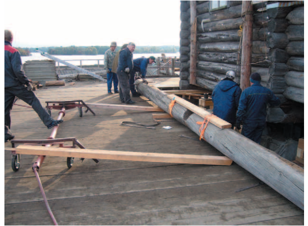
Fig. 23. Dismantling of 12-m long log from northern wall of the Church
