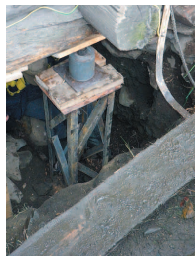
Fig. 34. Additional support during foundation pouring
