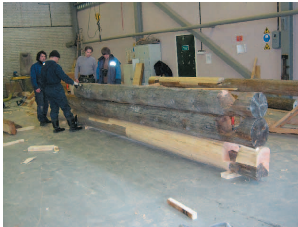
Fig. 14. Restoration of the Church refectory logs
