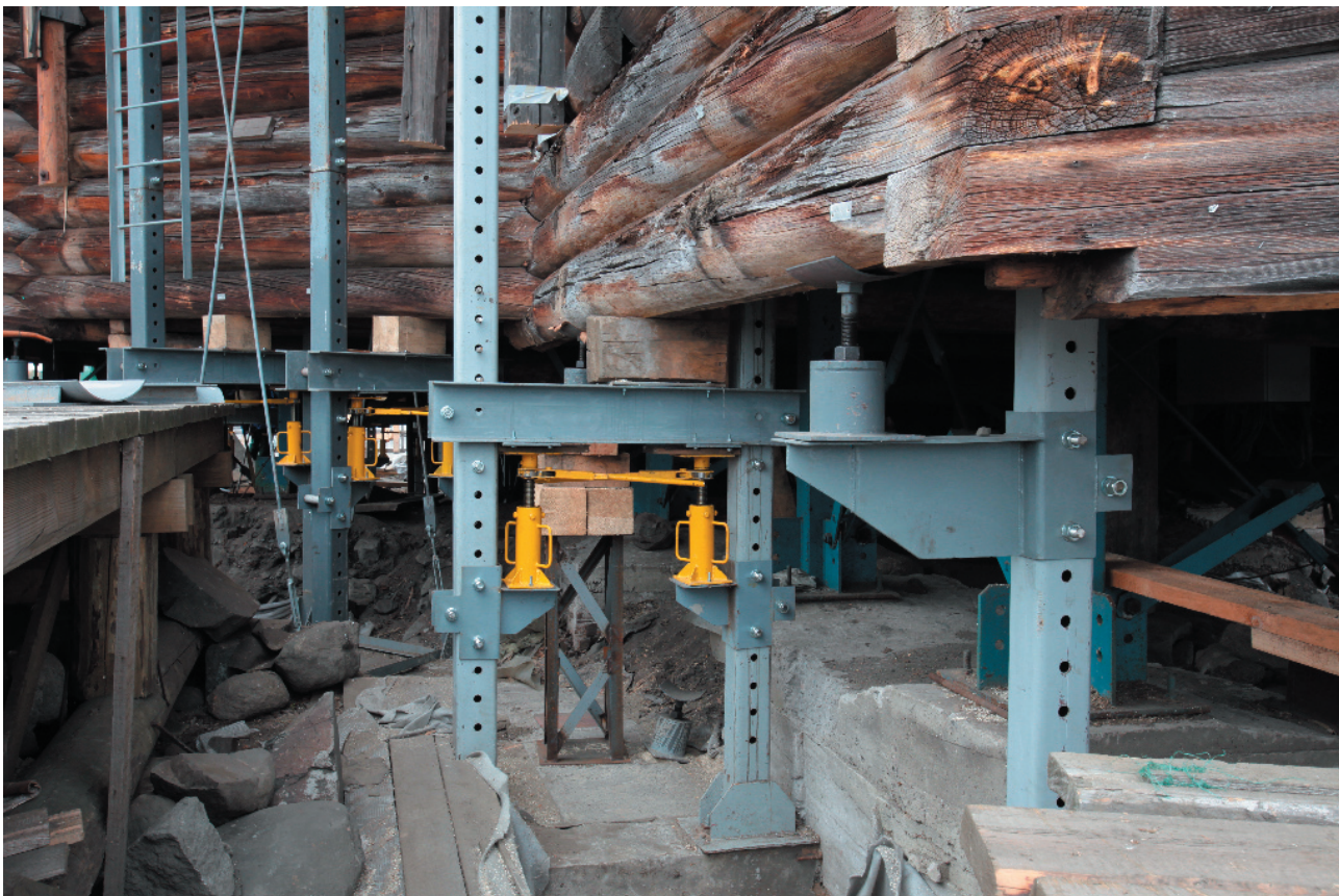
Fig. 15. Movable lifting mechanisms of lifting system: consoles, beams, jacks
