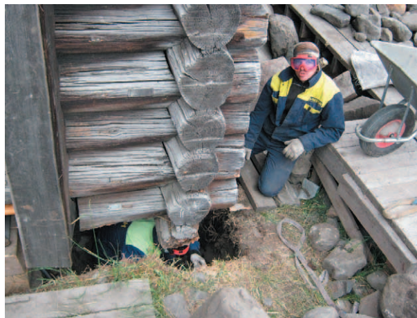
Fig. 10. Reconstruction of foundation
