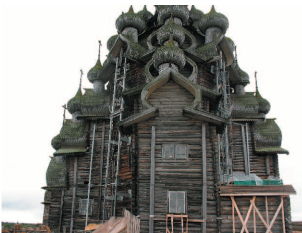
Fig. 11. External lifting uprights, general view from north
