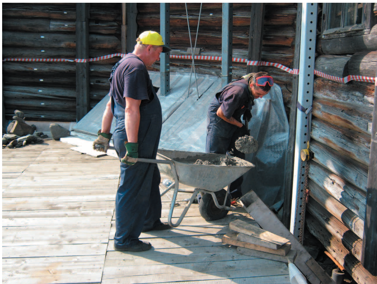
Fig.2. Pouring of lower part of rubble concrete foundation (underground part)
