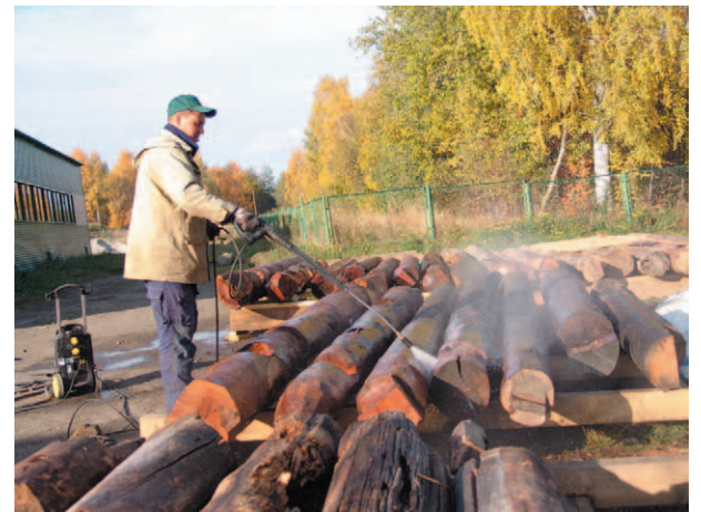
Fig. 27. Washing and air-drying of logs before stacking
