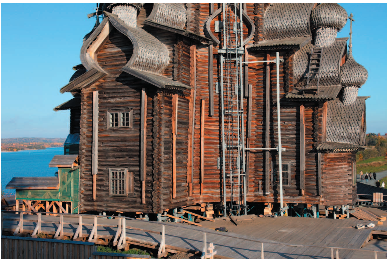
Fig. 20. General view of restoration workshop, lifting constructions and fragments of a dismantled restoration tier
