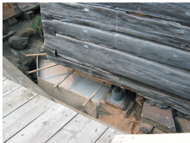
Fig. 32. Pouring of the underground foundation part in parts
