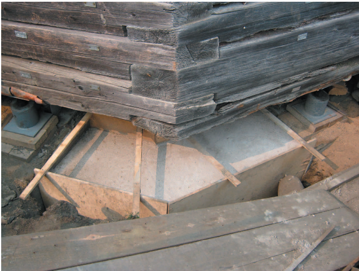
Fig. 3. Poured foundation in boxing; boxing is removed after 7 days of exposure
