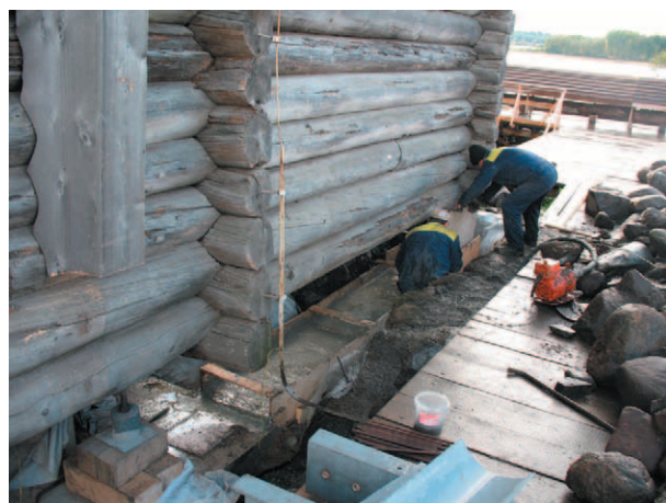
Fig. 33. Pouring of the foundation below lifted Church framework
