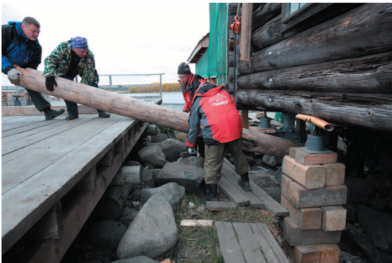
Fig. 14. Dismantling of beams, including 12-m long beams was done without difficulties
