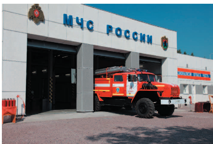
Fig. 3. Inauguration of the reconstructed office of the Karelian Division of the Ministry of Internal Affairs on Kizhi
