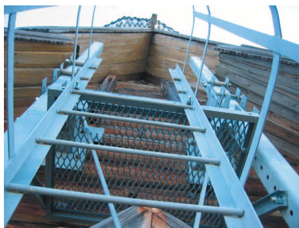
Fig. 21. Elongated posts mounted on diagonal Church log walls
