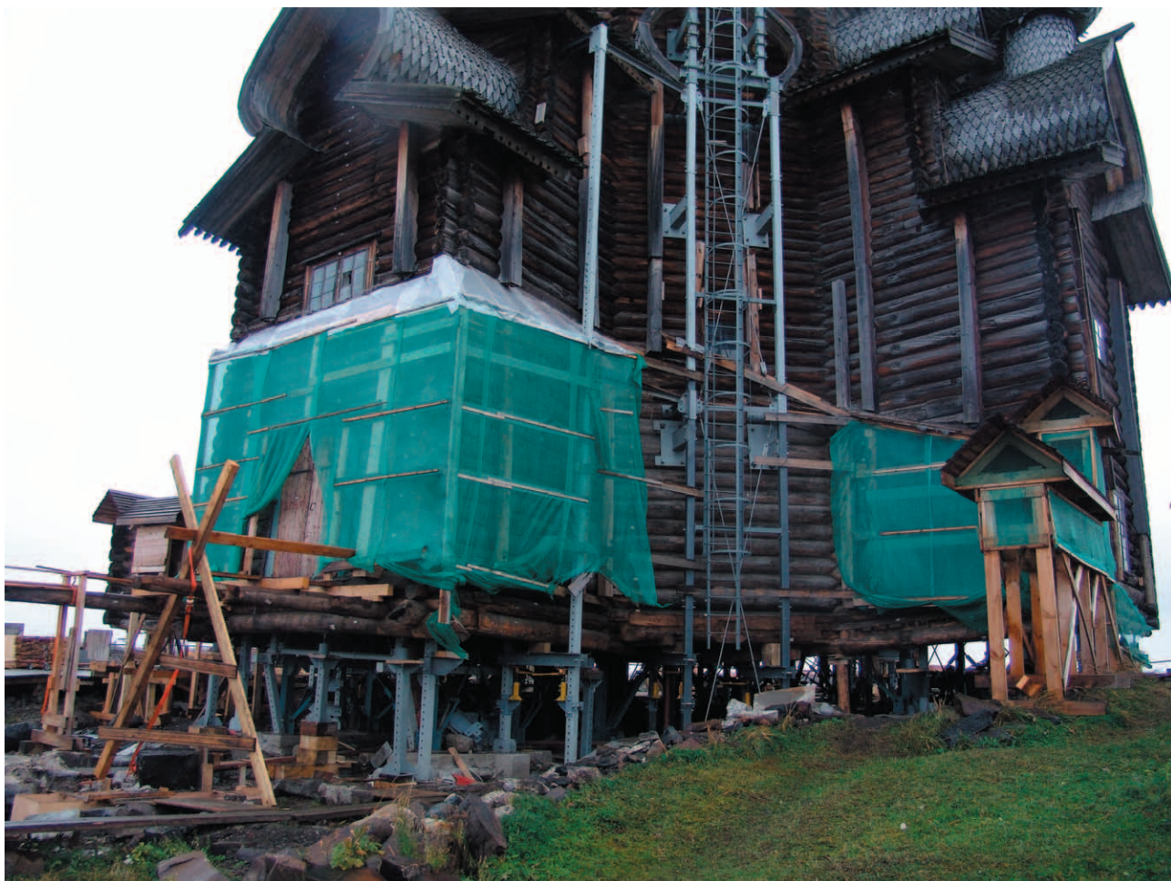
Fig. 16. Final stage of dismantling. General view.
