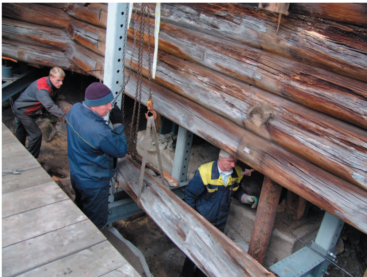
Fig. 6. Careful dismantling of logs, their placing on a site platform
