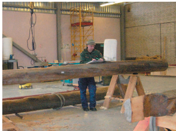
Fig. 18. Inspection and fixation of the refectory structural elements
