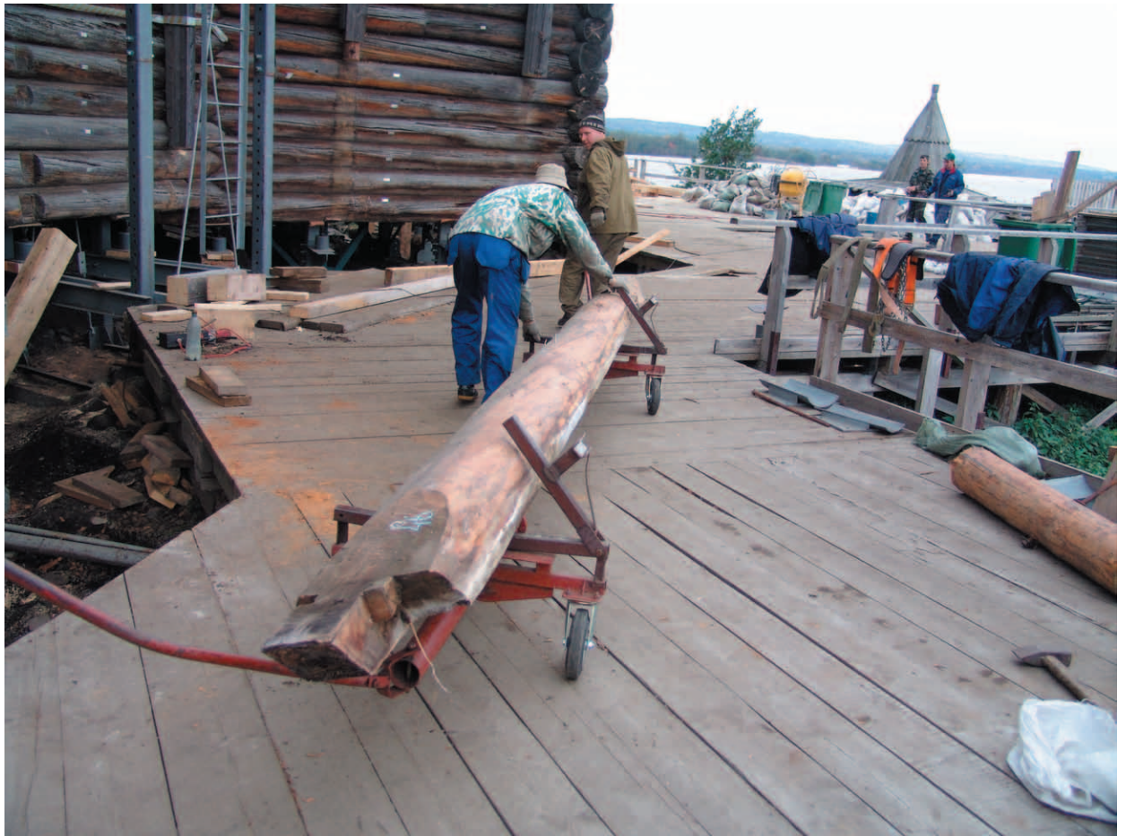
Fig. 7. Transportation of logs on a special transporting carriage to the temporary storehouse
