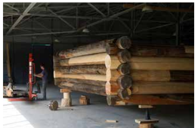
The test-assembly of the restored logs
