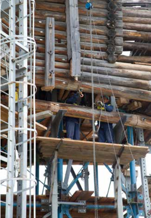
The disassembly of logs
